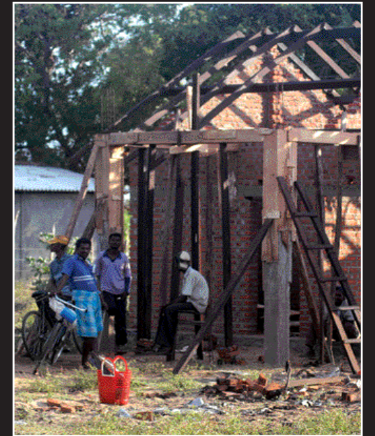
Re-construction of a house in progress
