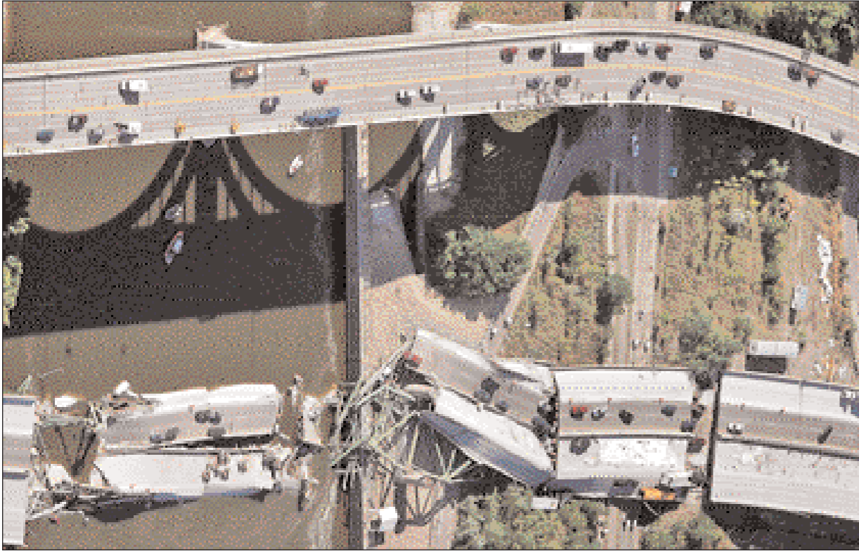
Minneapolis, Minnesota UNITED STATES: Vehicles rest on a collapsed section of the I-35W bridge August 2, 2007 in Minneapolis, Minnesota. Divers combed the dark, debris-strewn waters of the Mississippi river Thursday searching for up to 30 people missing after a major bridge collapsed at rush hour, killing at least four people. Officials expected the death toll to rise, with dozens of cars and trucks dumped in the river after massive sections of the eight-lane bridge roadway were sheared off Wednesday evening. AFP
