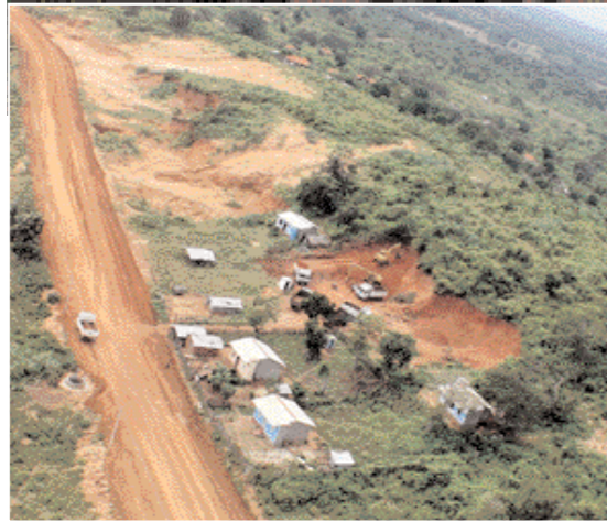
Developing road in Trinco
