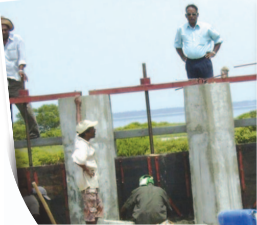
Work in progress of the salt water exclusion scheme in Jaffna
