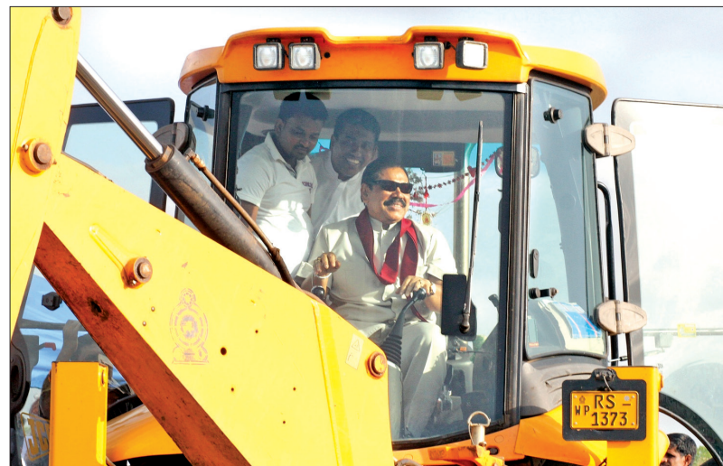
President Rajapaksa commissions reconstruction work on the Nikaweratiya, Magalle Wewa.
