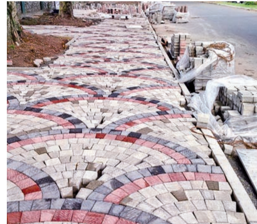
Pavements being laid
