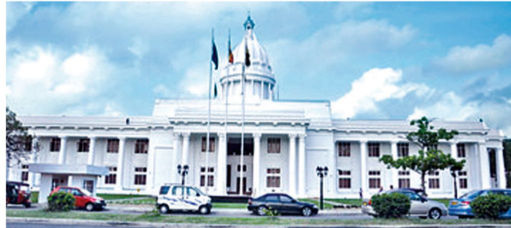
The roads around the Town Hall area
