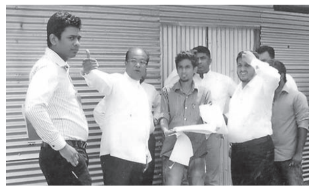
Puttalam Urban Council Chairman, K.A. Baiz inspects the construction work on the new auditorium of the Town Hall recently. Pic: M.U.M. Sanoon, Puttalam TKN Cor.
