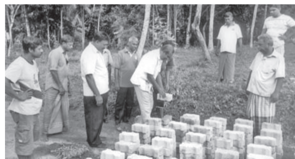
The inauguration program to lay carpet on the Ravi Tishan Road at Handapangoda in Ingiriya, organised by the Horana Pradeshiya Sabha was held recently, under the patronage of Chairman, Horana Pradeshiya Sabha, Yamith Chandana Hathurusingha. Here the Chairman launches the program.
