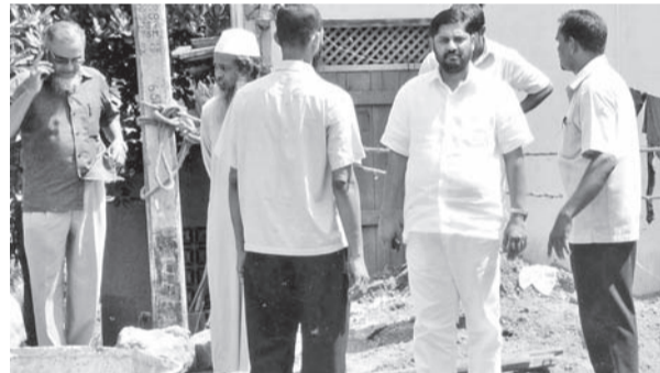
Western Provincial Councillor A.J.M. Faiz visited Zahira Vidyalaya, Hunupitiya, Wattala recently. Here the Councillor inspects the construction work on the new classrooms. Principal M.M.M. Kaleel and M. Fouzdeen are also in the picture.
