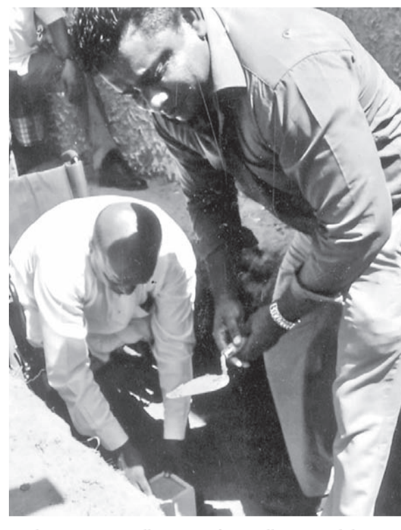
Work on a parapet wall at a cost of one million around the Panadura, Ambalanduwa Muslim Vidyalaya was inaugurated recently. Here Western Provincial Councillors M. Amjad and Ranaviru Wikum Gunasekara lays the foundation stone. Pic: M.S.M. Munthasir, Panadura Central Gr. Cor.
